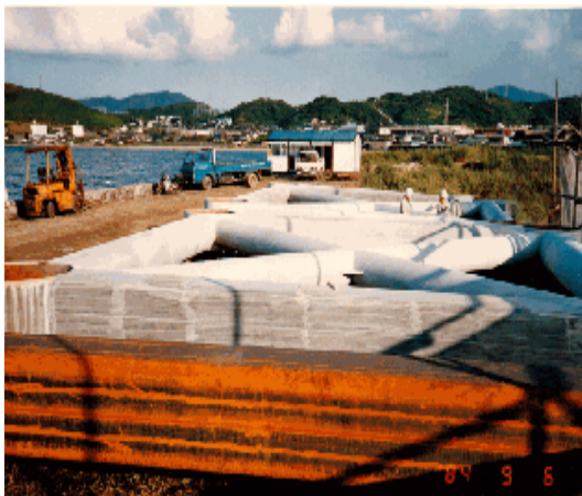
Diagram 8 Coating on joint part
