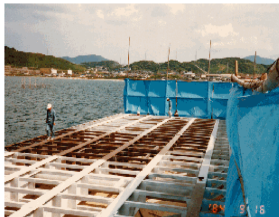
Diagram 9 Setting subfloor slab of beam and pier
