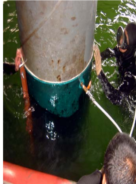
Diagram 17 Removing water from the formwork
