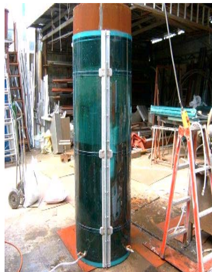
Diagram 15 Closing formwork on land
