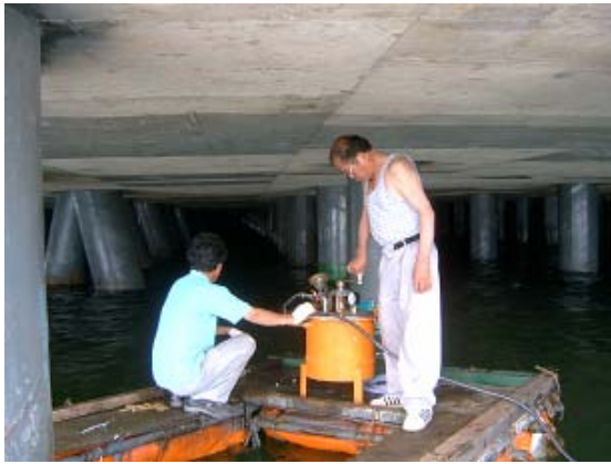
Diagram 4 Injection of Mighty CF-CP
