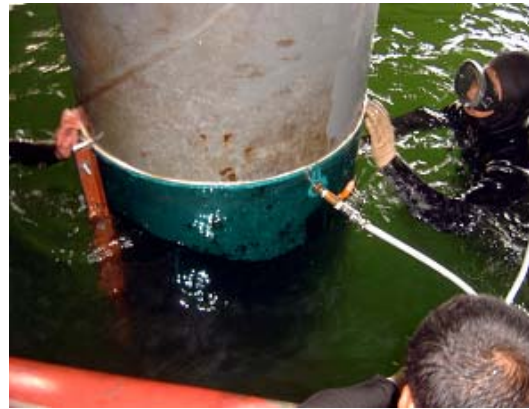
Diagram 5 Confirmation of exhaust at top vent holes
