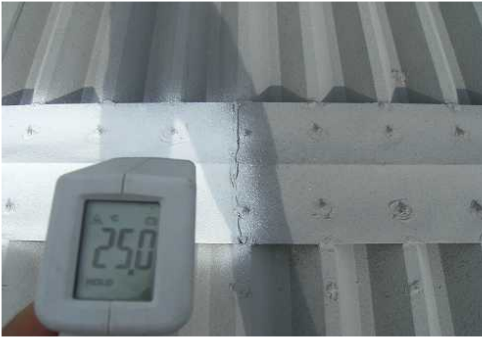
Temperature of Roof(Sun Guard finish on Mighty CF)
