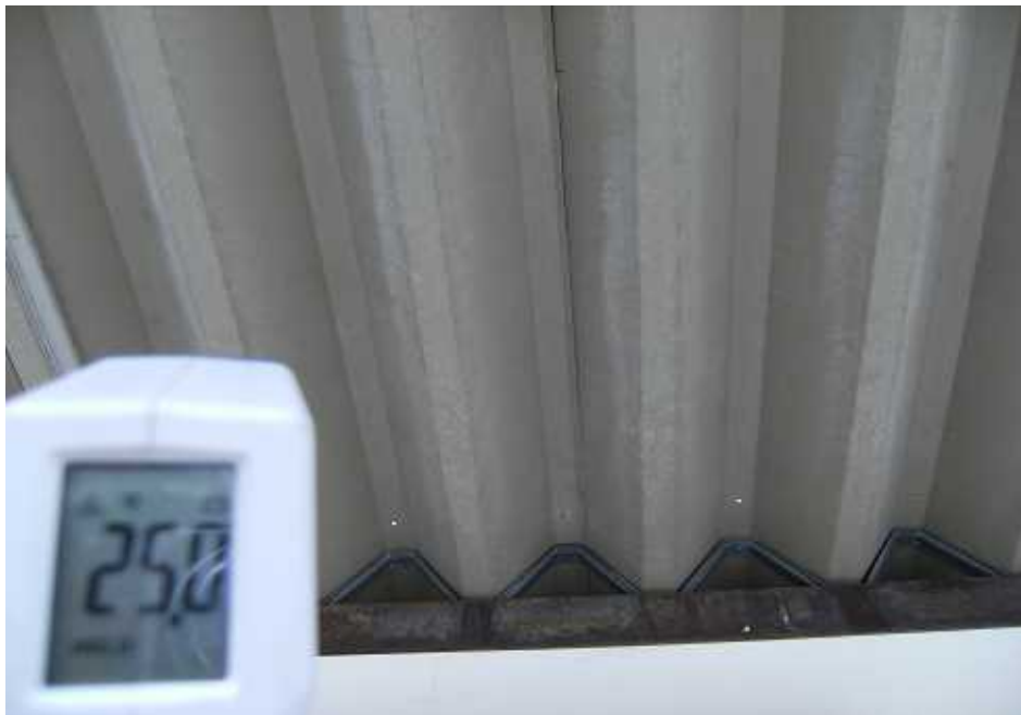
Temperature of under the Roof
