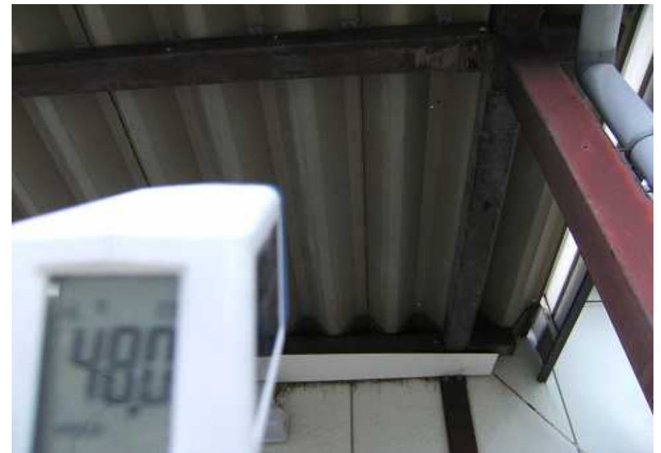
Temperature of under the Roof
