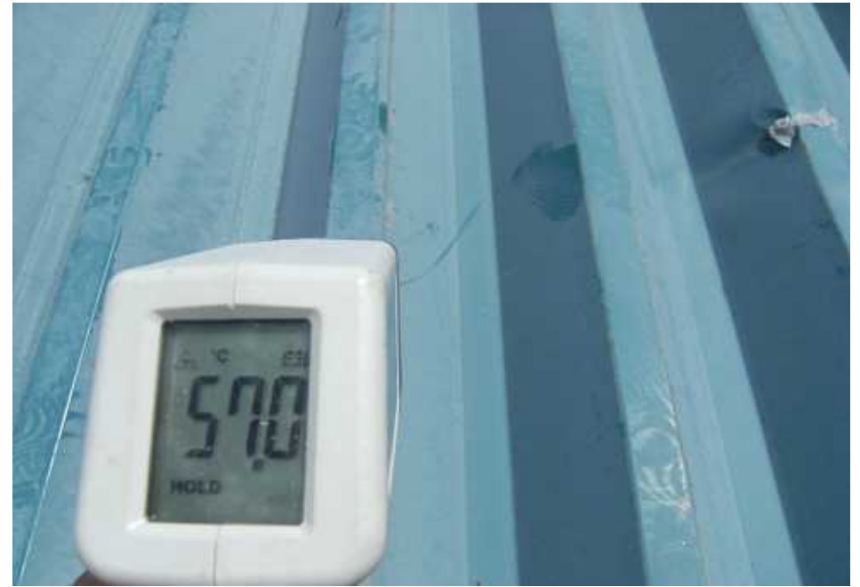
Temperature of Roof 57 AM 10:00
