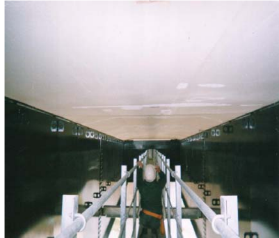
Photo 18 Mighty Coat CF-CP coating of Kurigaya Viaduct under slab
