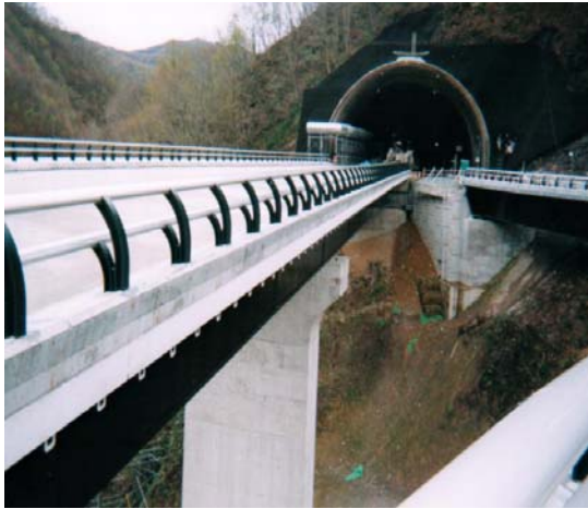
Photo 17 Birds eye view of the Kurigaya Viaduct
