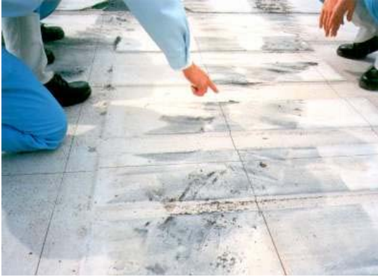
Photo 15 Inspection after the zigzag driving test
