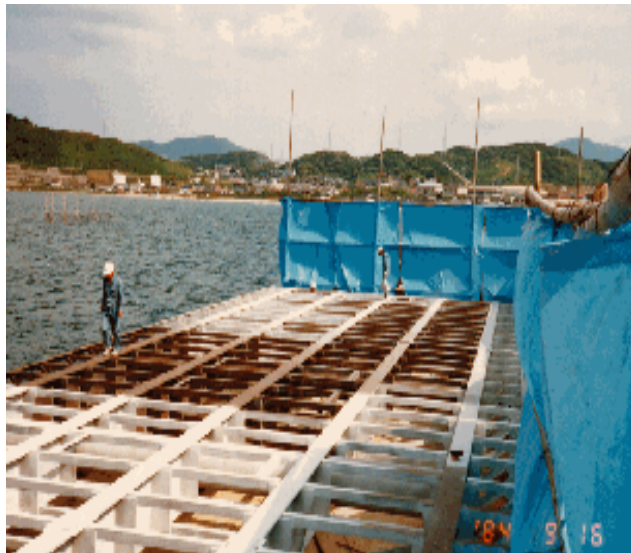
Photo 4 Beam structure of Pier
