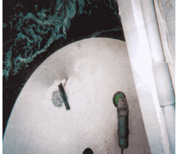
Photo 7 After grinding top coat
