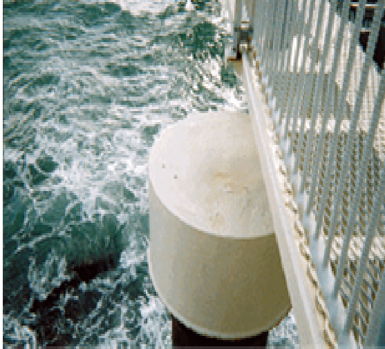
Photo 6 Top of steel pile
