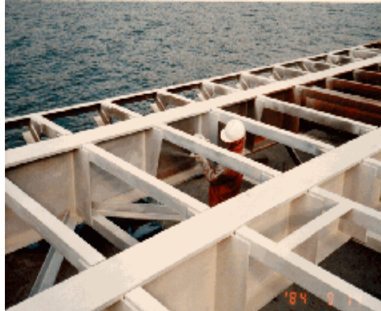
Photo 5 Spraying of Mighty Coat CF-CP
