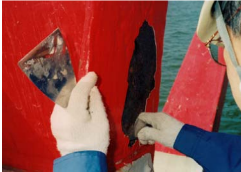
Photo-3 Removal of Fluorine Resin coating layer
