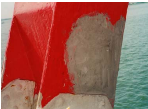
Photo-7 After repainting with Mighty Coat CF-CP
