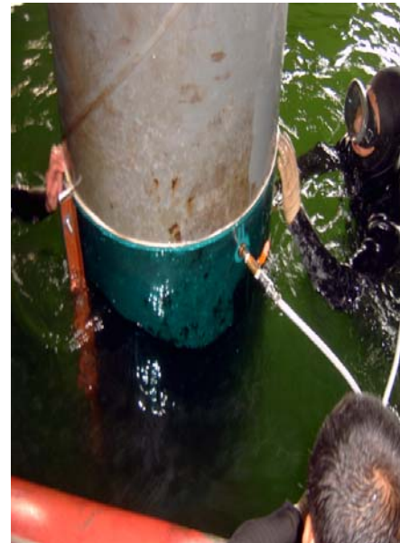
Diagram 17 Removing water from the formwork
