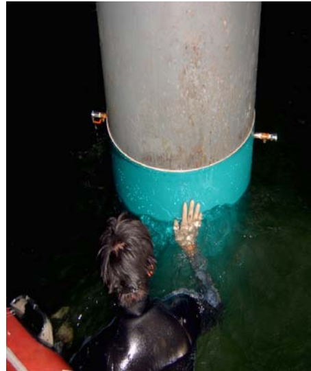
Diagram 19 completion of injection
