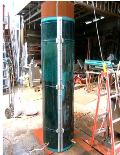
Diagram 15 Closing formwork on land
